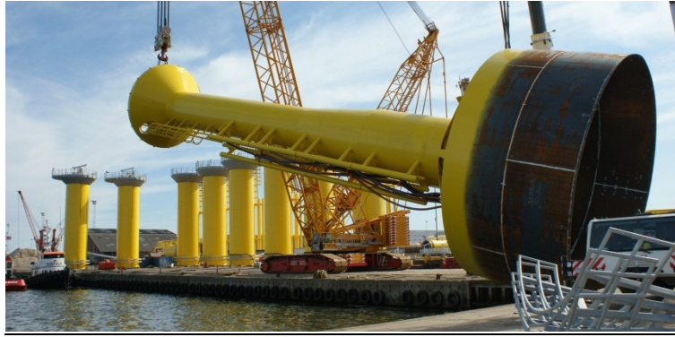
Figure 66: Bucket foundation of a mobile met mast for the OWF Horns Rev 2 during erection in the port (source: LEBLANC et al. 2009)
