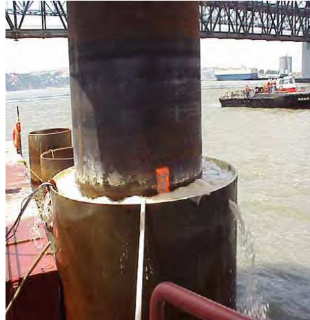
Figure 16: Isolation casing with additional bubble curtain between pile and isolation casing during piling of a 2.4 m pile at the Benicia-Martinez Bridge, California (source: CALTRANS 2007)
